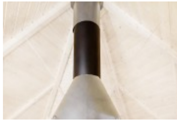
Grill Chimney Extension
